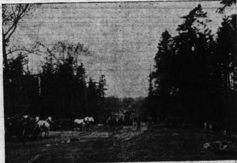
AT WORK ON PART OF SHORE ROAD, "UPLANDS"
